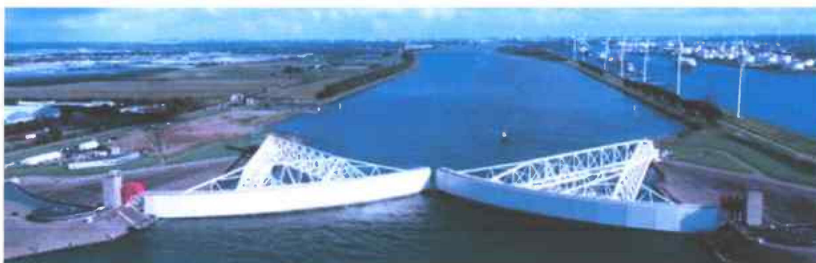
Figure 5-2 Svingbare porter utenfor Rotterdam
